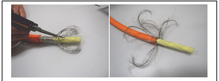
Fig. 8-5: Split the shield braid open
